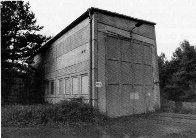
Engine shed (2 on the site plan). Photo Tim Robinson
